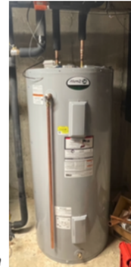
AO Smith Model LTE 119 gallon hot water tank with two 4.5 kW elements
